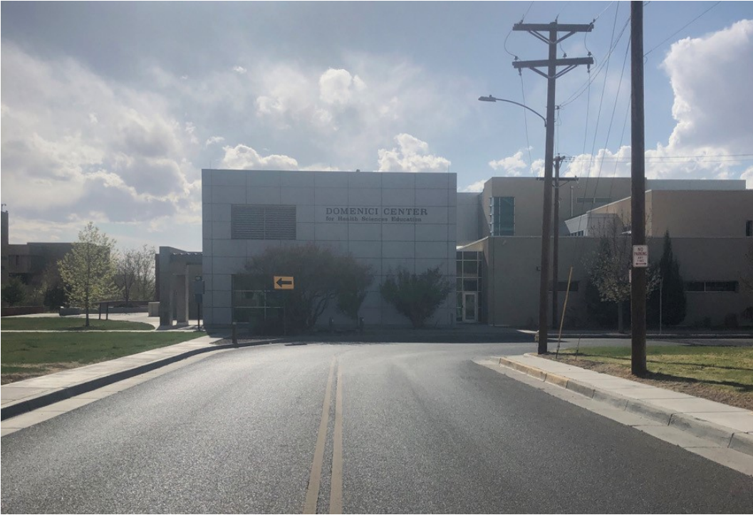
Figure 4: Marble Avenue Road Looking West
